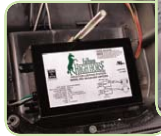
Complete Ballast & Lamp Mounting Assembly
