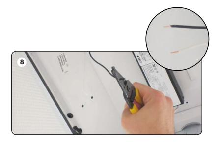
**STEP 8:** Prepare input power by stripping input power leads 1/4". See **Figure 8.**
